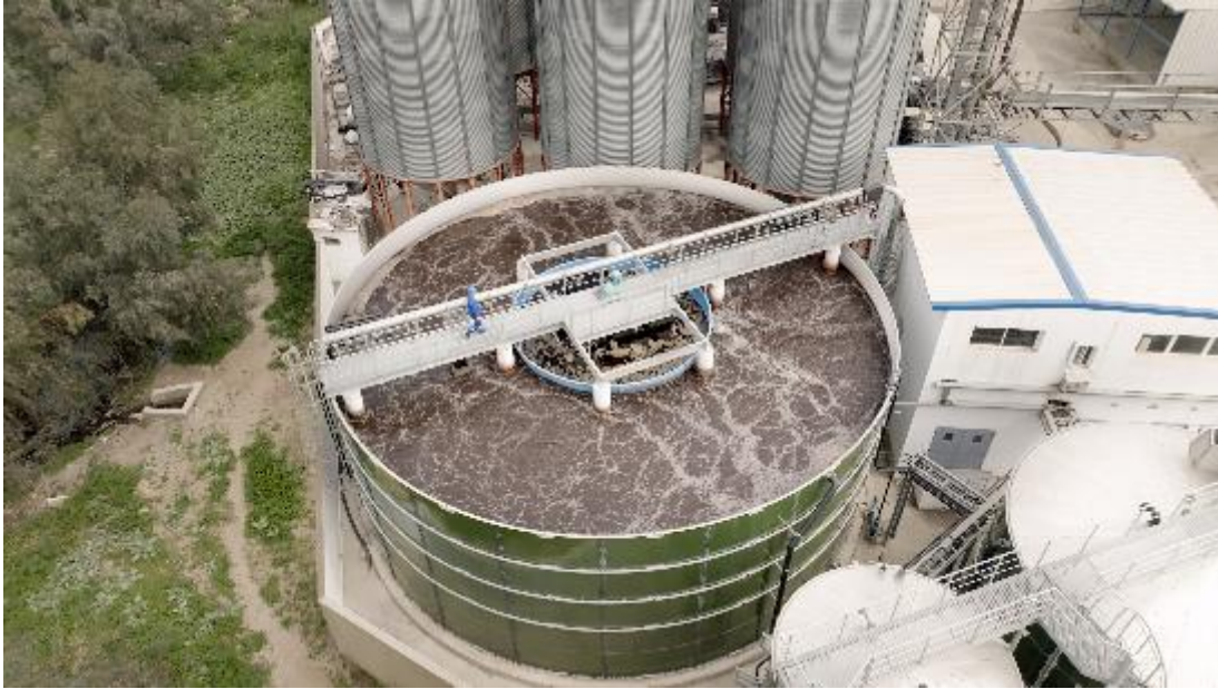
Image: An aerobic treatment plant at Bioresine treats the wastewater from the production of active pharmaceutical ingredients for direct discharge and saves space, too.
